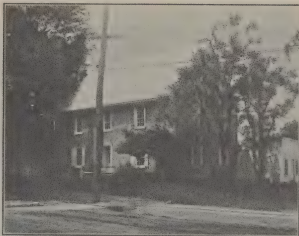
This finest of the early Moravian houses stood at the N. W. corner of Main Street and Keystone Avenue. It was built in 1763, no doubt by Sebastian Knauss who owned the lots. According to tradition it was used as a schoolhouse for a time. Later known as the Everitt house (Thomas Everitt had married the granddaughter of Sebastian Knauss), and still later as the Walter house, it was demolished about 1914.
